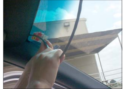
View of DB-25 cable, under headliner, heading toward control head.
